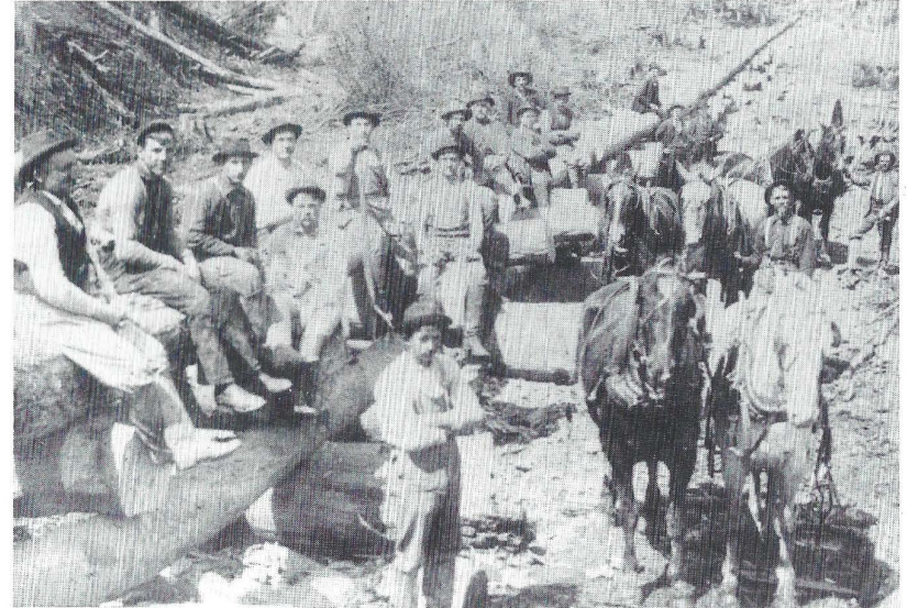
Teamsters who drove the horse teams hauling timber are shown at the Stull log slide. Logs loaded on the slide descended by gravity to a rail site for shipment to the mill. A log slide could also carry logs directly to a mill pond. Noah McCloskey, the woods boss, is the first man on the left.
