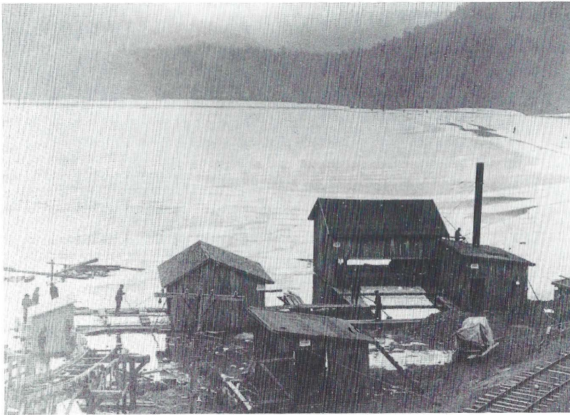
At No. 2 Dam, the first mill is at the right rear, the second mill is in the center, and the kicker house is at the left.
