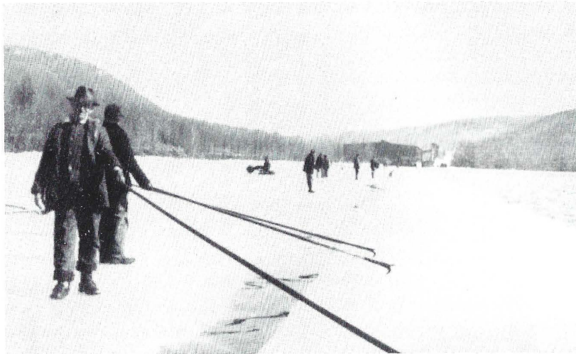
Two workmen pause for the photograph. With a pike pole, they can push a raft of ice down the channel to the mills and ice plant at Dam No. 2. As the rafts approach the mills, they are spudded apart into 13.8 by 12.4 foot floats.
